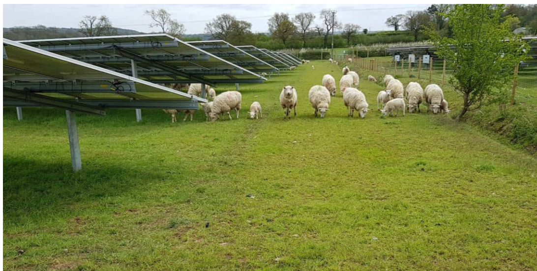
Figure 2-14: Sheep grazing on a solar PV facility
