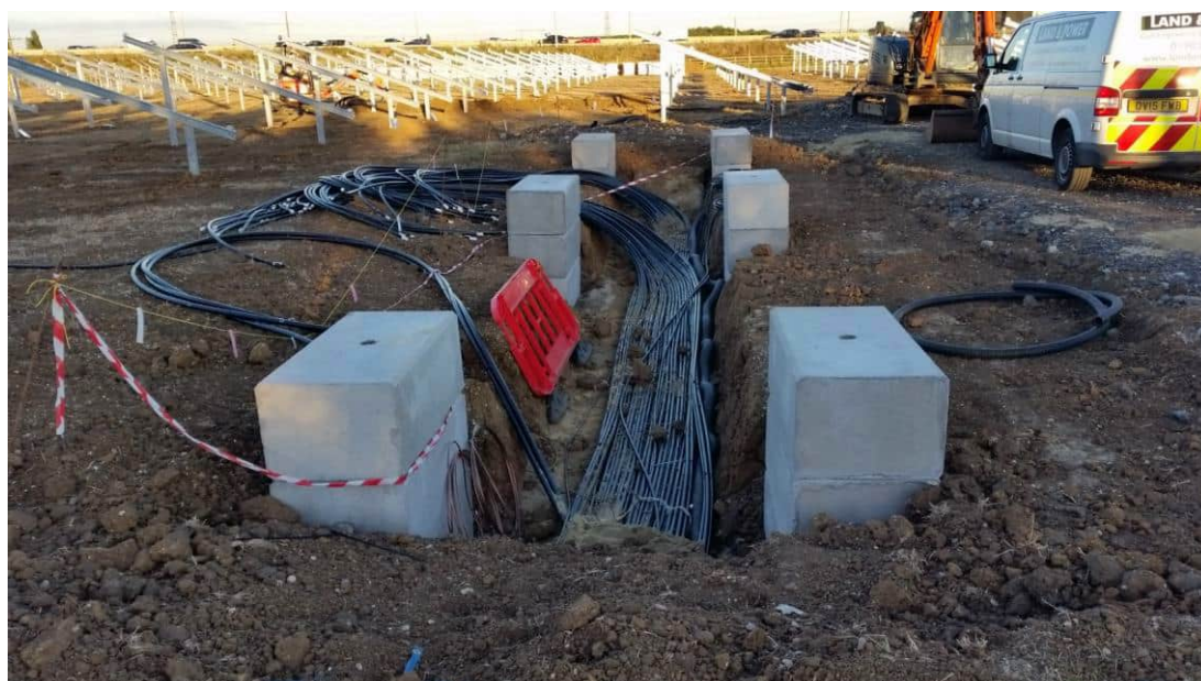
Figure 2-9: Example underground cable installation
