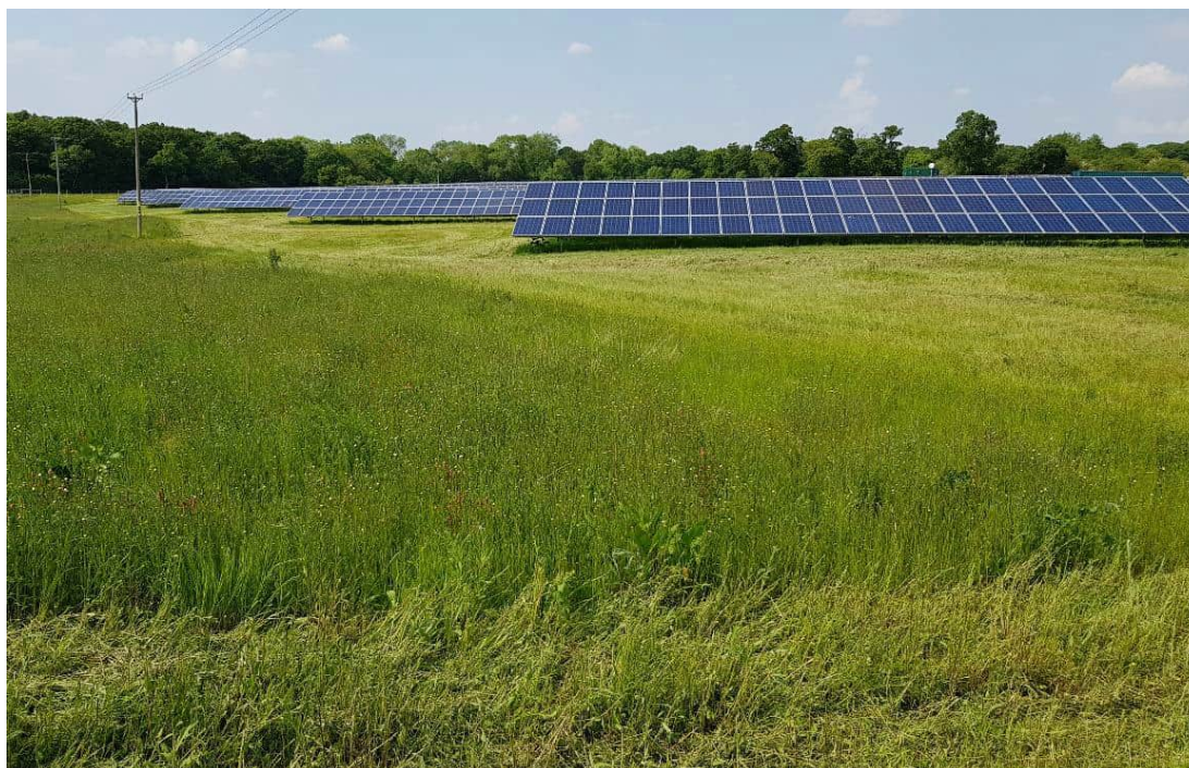
Figure 2-13: Landscaped solar PV facility
